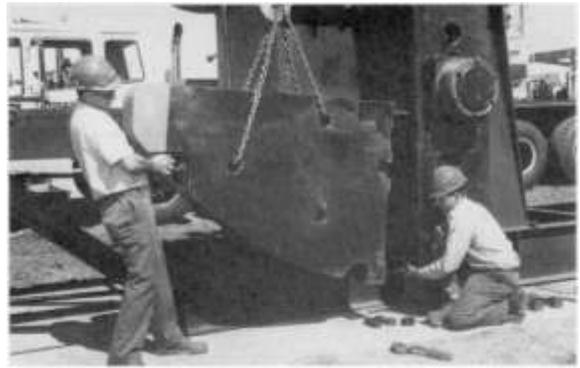
**Step 5:** Install a flat washer, a standard nut, and jam nut on each of the counterweight bolts and tighten securely.
