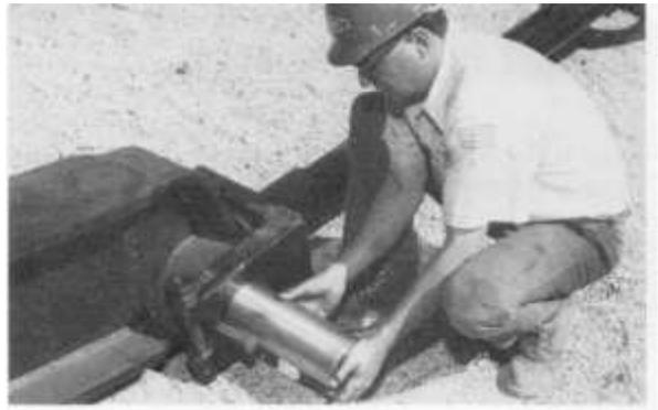
**Step 5:** Connect the lubrication line from the pitman arm to the equalizer, and from the equalizer bearing, using the flexible hoses provided in the parts box.
