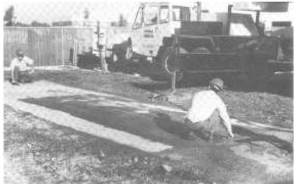
**Step 2:** Refer to the LS foundation plan furnished with the unit to determine the specific distance your pumping unit should set from the well head. Measure the distance from the wellhead and mark a line that intersects with the centerline.
