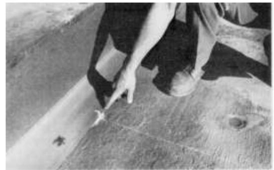
**Step 7:** Place a level on the base beams to determine if the pumping unit is setting level. Level the unit as the foundation requires.
