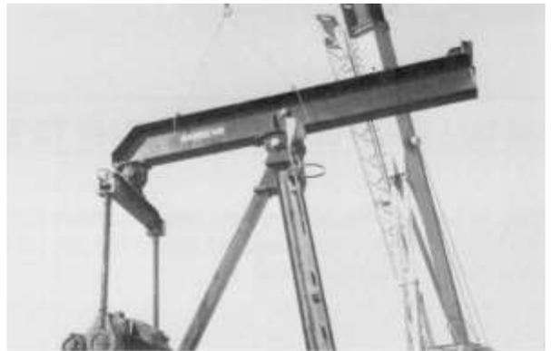
**Step 2:** Position the center bearing housing on top of the samson post. Insert the bolts and hand tighten.
